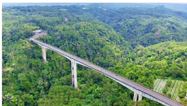
Figure 2. Tukad Bangkung Bridge, Pelaga Village (Taken by Urbanasia, 2019)
