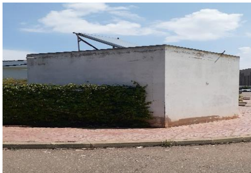
Figure 1. Picture of the studied cell (building)
