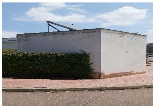
Figure 1. Picture of the studied cell (building)
